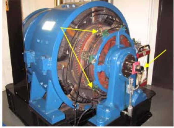
Photos #21 & #22 – Examples of electrical shock hazards associated with elevator drive motors. On the right most photograph, note also the encoder (yellow arrow).
