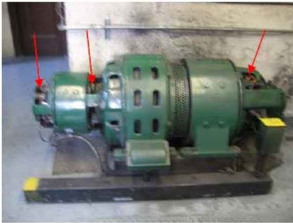
Photos #25 & #26 – Examples of elevator motor generator sets and the potential for electrical shock hazard associated with each.
