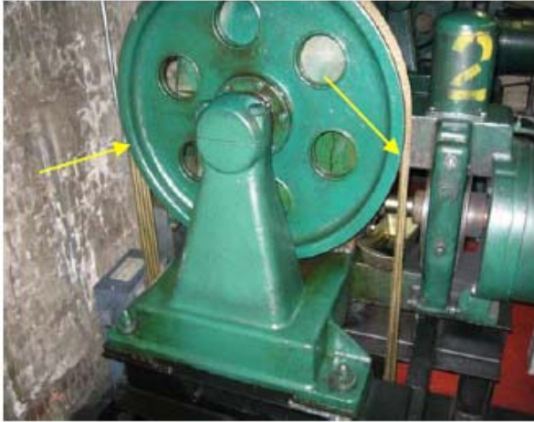
Photo #1 – Worm gear traction sheave
