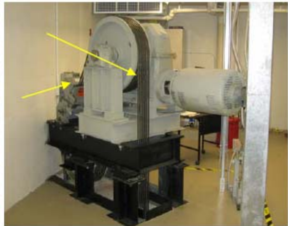
Photo #2 – Overhead geared traction machine
