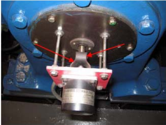
Photos #23 & #24 – Examples of encoder and tachometers as mounted to elevator drive machines. The tachometer as shown in the right most photo is a close up of the unit as shown in Photo #3,
