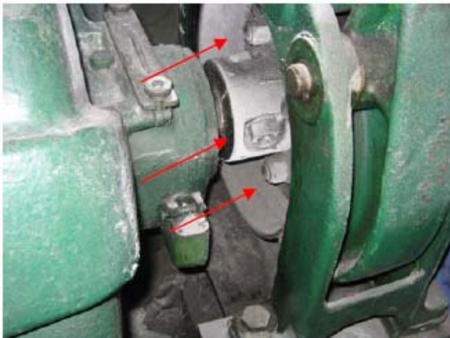
Photo #15 – Coupling fitting used to connect motor drive shaft and machine brake pulley.
