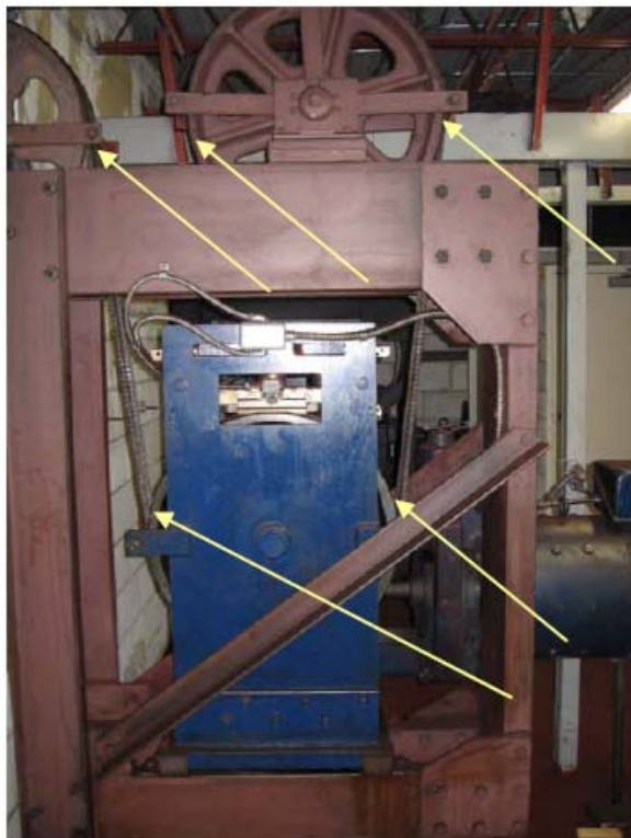
Photo #10 – Offset Traction Machine with deflector sheaves
