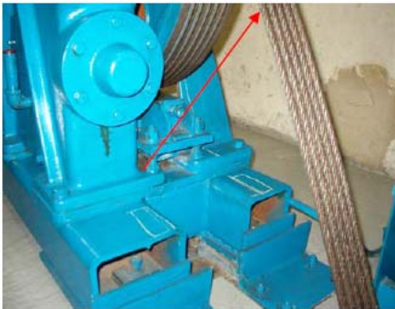
Photo #7 – End shot of typical geared machine
