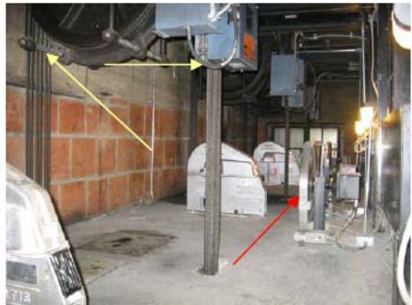
Photo #8 – Secondary level showing deflector sheaves (black color wheel), rope gripper (light blue color box, car position unit (red color arrow) and car governors (silver objects, which you will note are fully enclosed).
