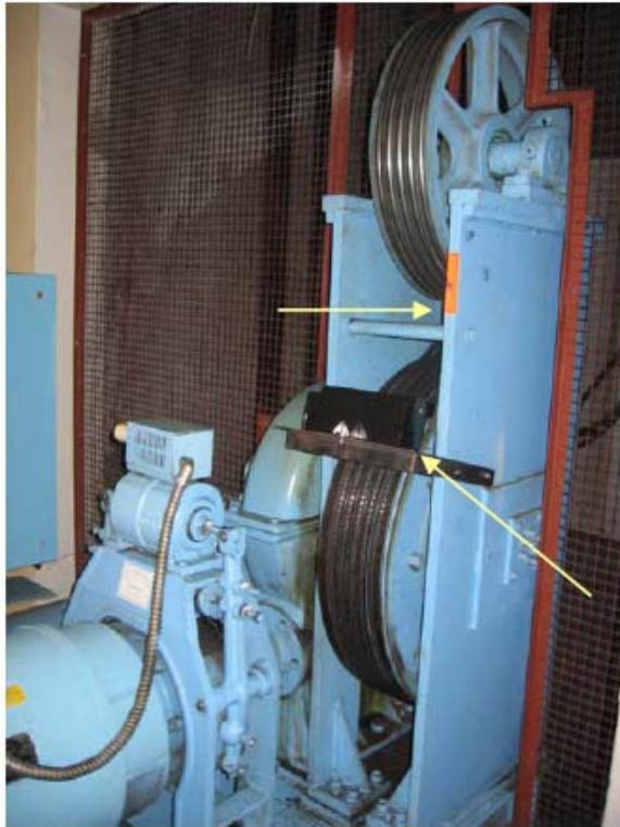
Photo #9 – Basement Traction Machine with deflector sheave
