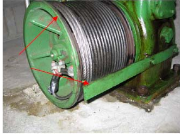
Photos #5 & #6 – Overhead drum drive machine. Suspension rope coils around the drum or unwinds off the drum, depending upon car direction of travel. Used for dumbwaiters, older small capacity freights, and very old small capacity passenger elevators. Note, open end of electrical motor, potential shock hazard.
