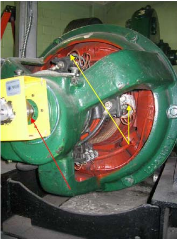
Photos #19 & #20 – Examples of electrical shock hazards associated with elevator drive motors.
