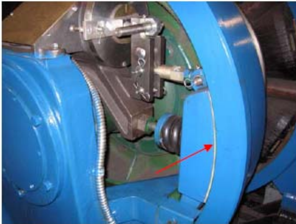
Photos #17 & #18 – More examples of elevator brakes, used on gearless traction machines.
