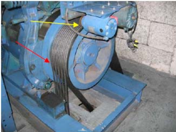
Photos #3 & #4 – Overhead gearless traction machine with tachometer/encoder shown in left hand photo (see also Photo #24), and close up of drive sheave shown in right photo.
