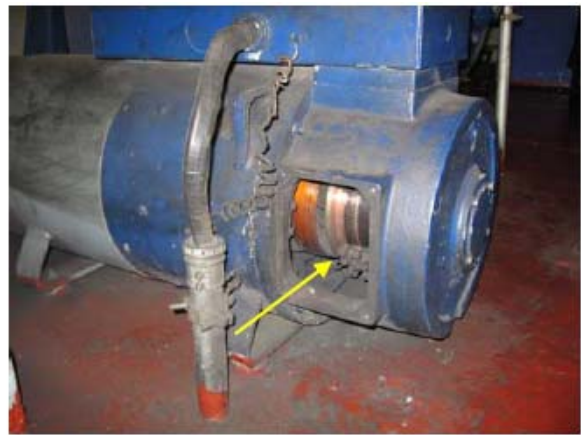
Photos #25 & #26 – Examples of elevator motor generator sets and the potential for electrical shock hazard associated with each.
